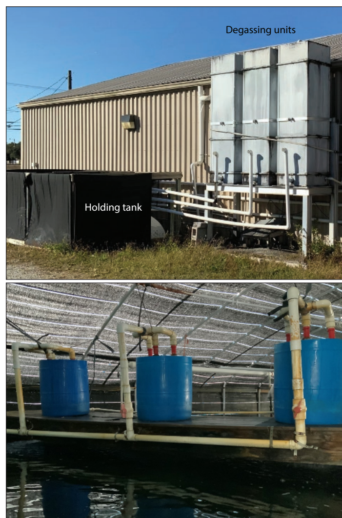
Figure 6. Two different setups showing the combination of degassing units and holding tanks, which could also include biofiltration. At top, pipes take water from the degassing units to the storage tank. At bottom, the water falls directly from the degassing units (blue barrels) into the holding tanks below.
