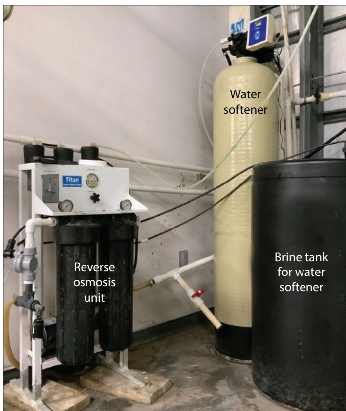
Figure 5. Reverse osmosis unit and water softener components at the Tropical Aquaculture Lab of the University of Florida Institute of Food and Agricultural Sciences. After the water passes through these components, it is stored in a 1,500-gallon storage tank for later use.
